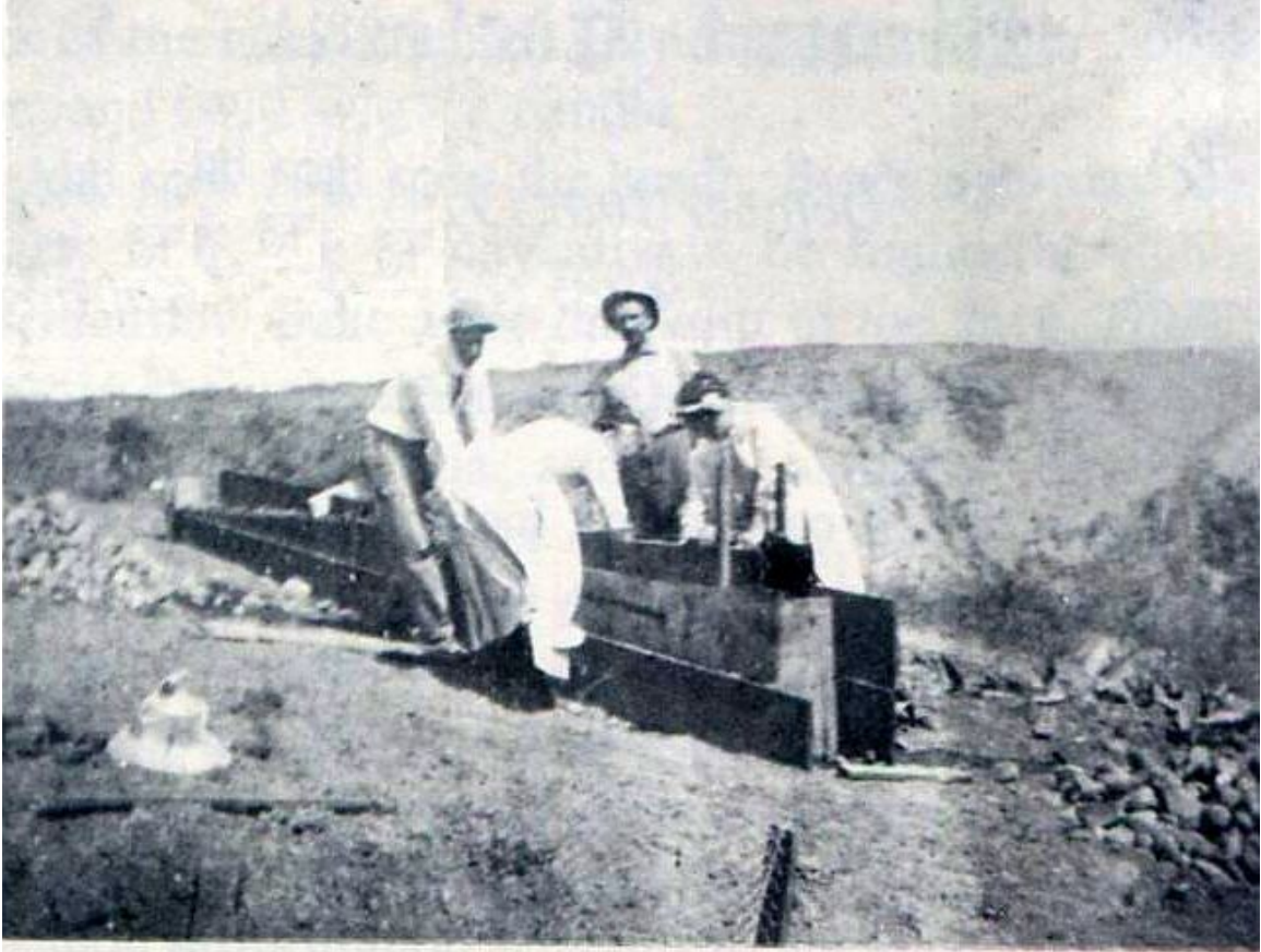
LAYING OF FOUNDATION FOR FIRST COTTAGE
